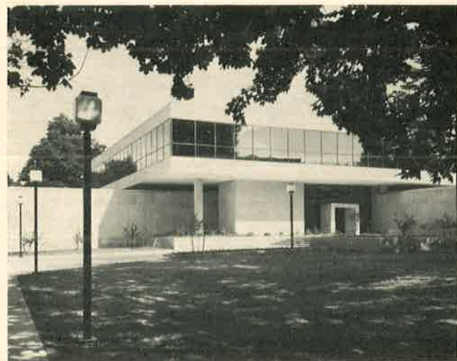
County Office Building Entrance
