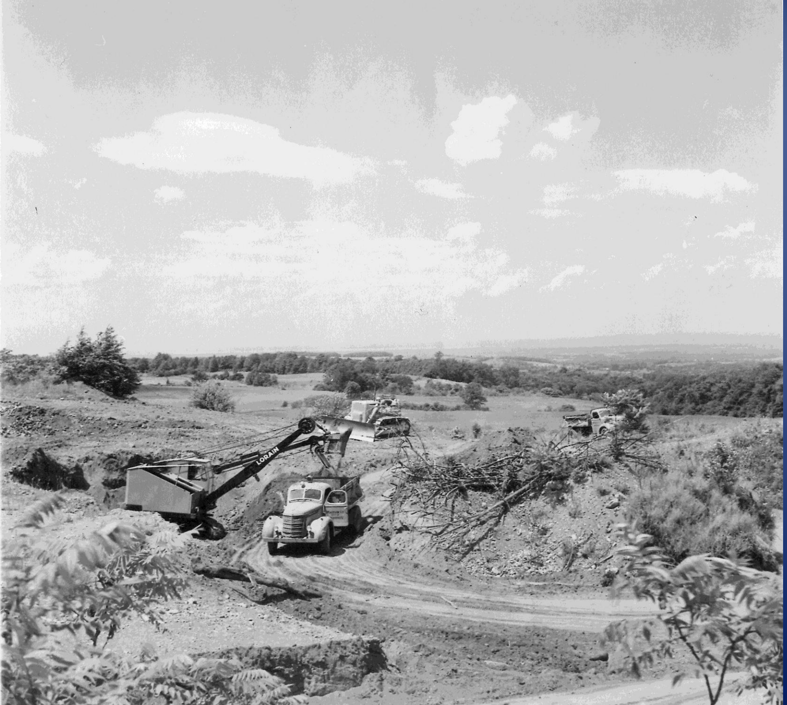
Eddy's gravel bed in regrading mile on the Buyea rd. July 2nd 1953
