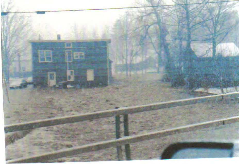
Oneida Creek Flooding- Normal creek bed is right of two story building. View looking south from bridge on Valley Mills St.
