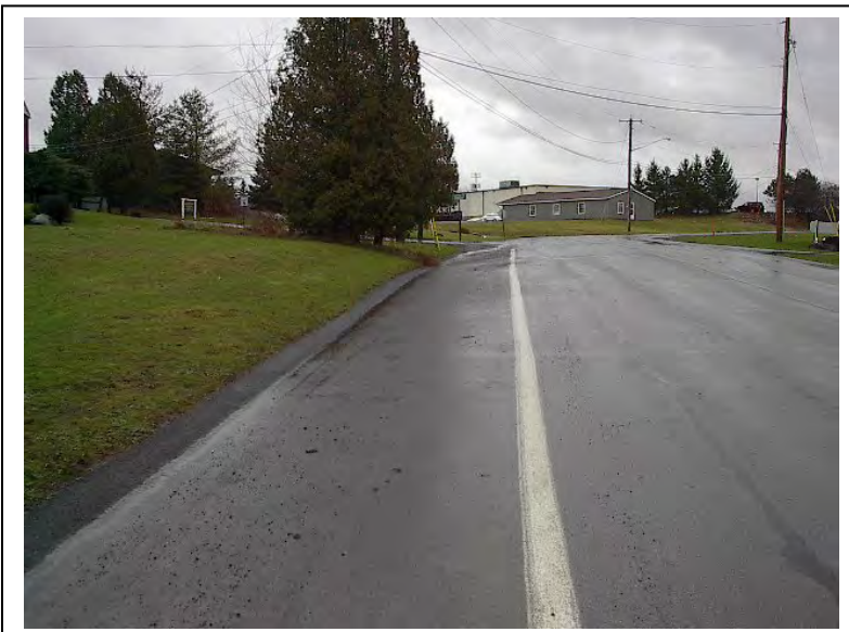
Paved Road Shoulder of Carriage Lane.
