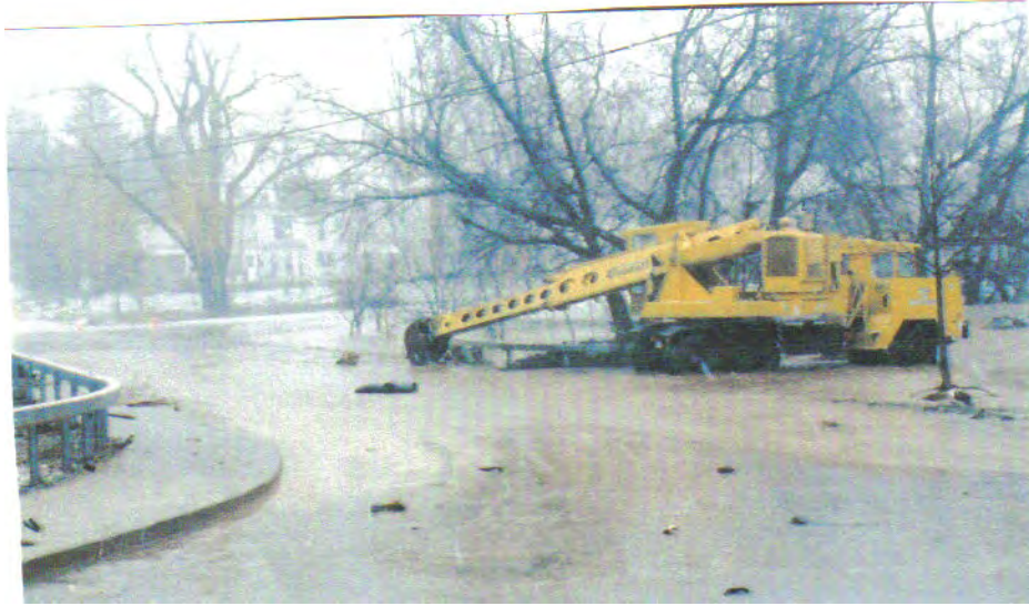
Highway Department Gradall clearing debris from culvert on Valley Mills Rd.
