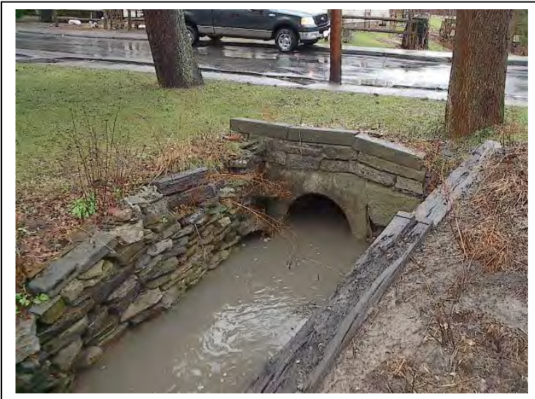
Culvert outlet at Burr Street Outlet Ditch.
