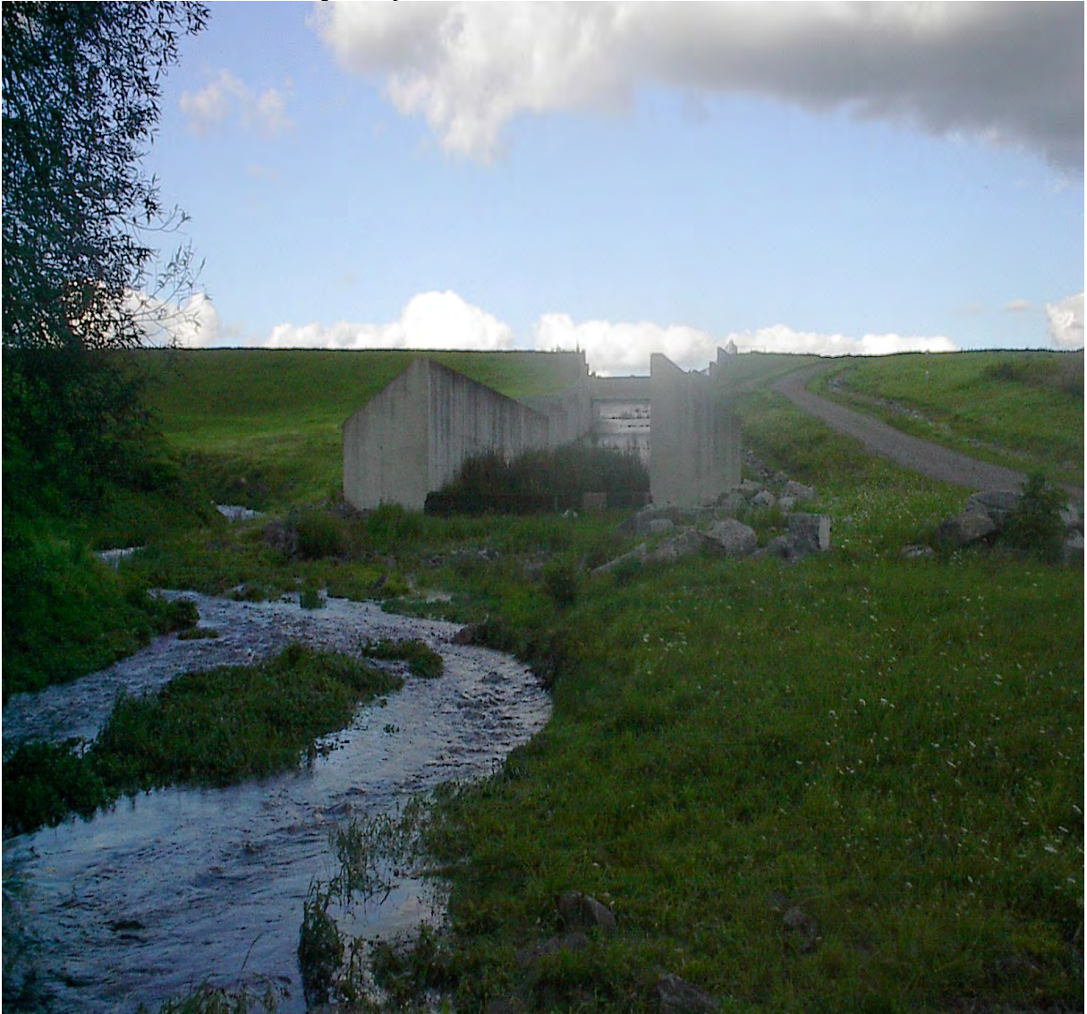
Newly constructed spillway for Lake Moraine.
